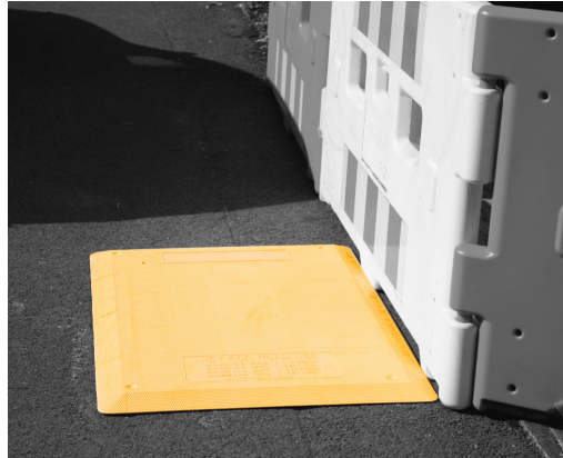
TRENCH COVER INSITU
