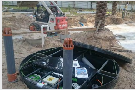
▶ Treatment plant during installation.
