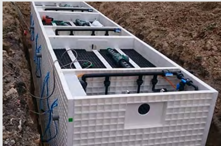
▶ Treatment plant during installation.
