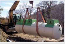
Each wastewater treatment plant is constructed of lightweight SMC and is easy to manoeuvre which simplifies the installation process.
