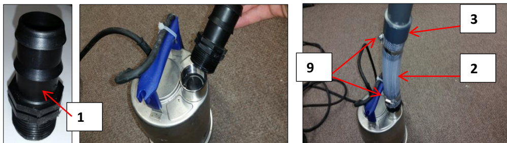
Figure 12 Fitting pipework to Pump.
