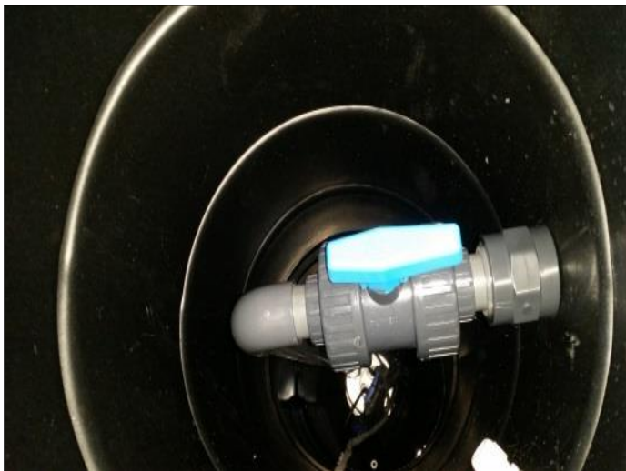
Figure 14 Pipework, assembly inside Pump Chamber.
