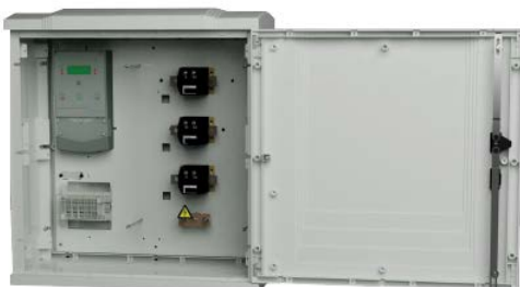
Example: electrical indirect metering
